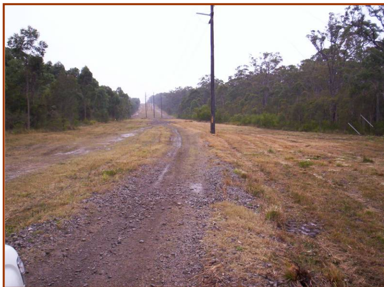
Photo 16 – Surficial filling along transmission easement (looking north-east Lot 96)
