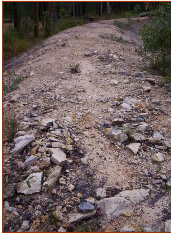
Photo 8 – Clays/siltstone within dam wall (looking east Lot 95)
