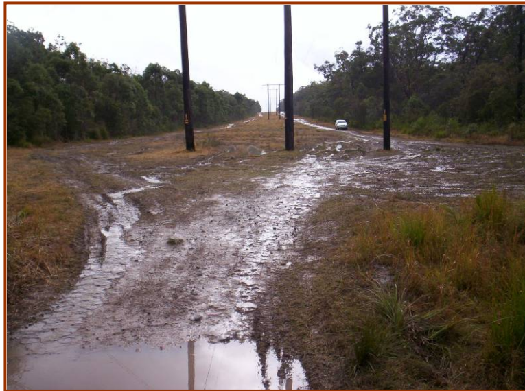
Photo 7 – Minor soil erosion within transmission easement (looking north-east Lot 96)
